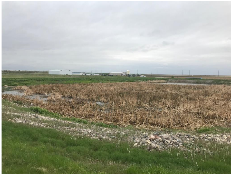
Figure 1—Lagoon Pond Cell #1, Looking Northeast
