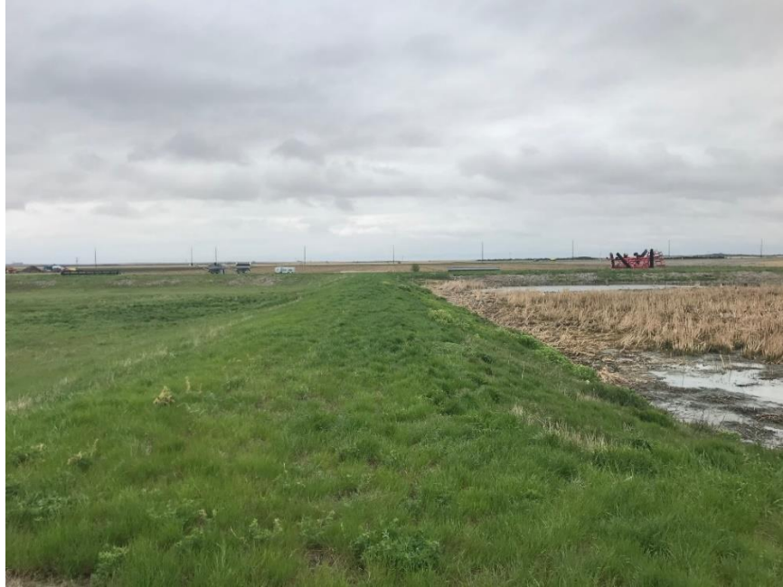
Figure 2—Berm Separating Pond Cell #1 and #2, Looking East
